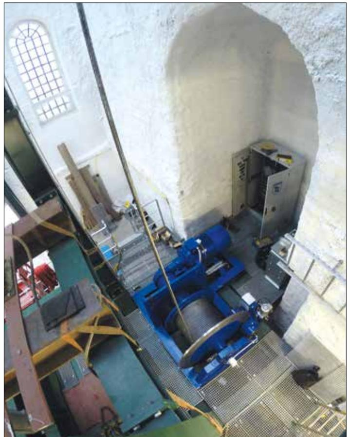
**SB-E 316 as a hoist winch for a pump line**
