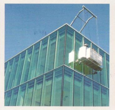
Freestanding roof car Fully balanced trackless compact unit, traversing on a load bearing concrete runway
